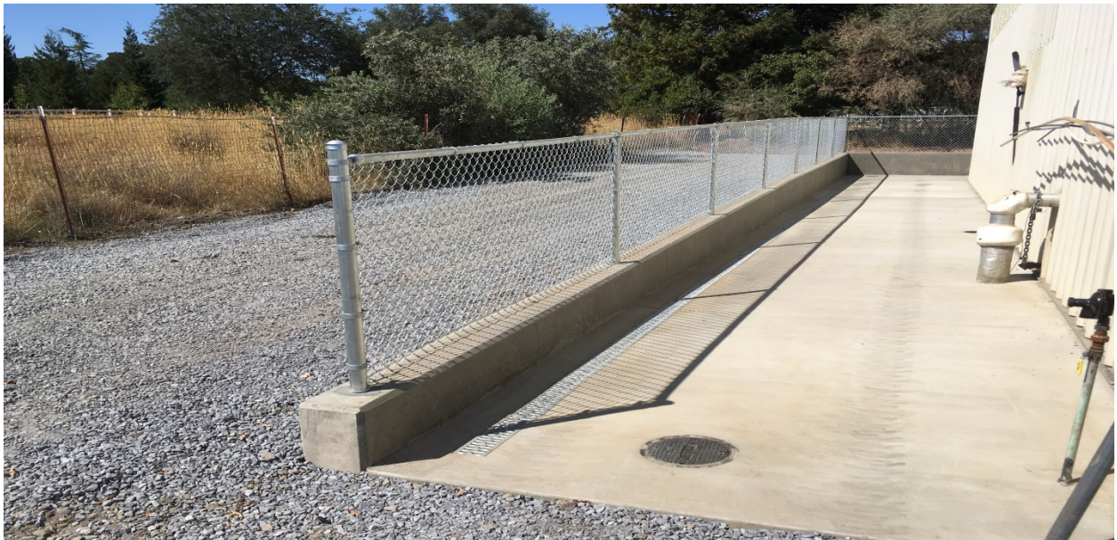
New Retaining Wall & Drainage Improvements
