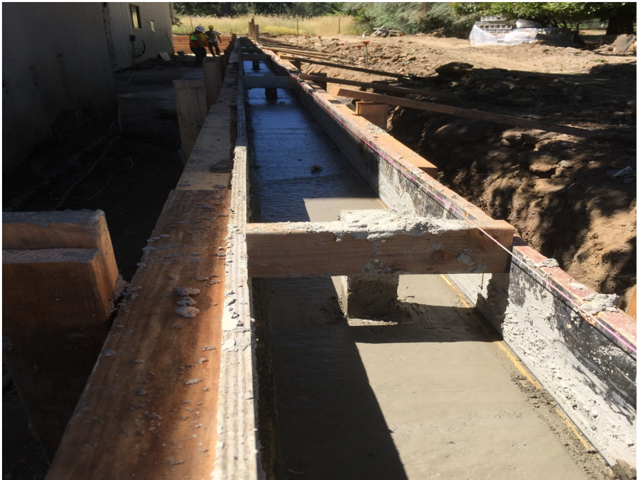
Pouring the Retaining Wall
