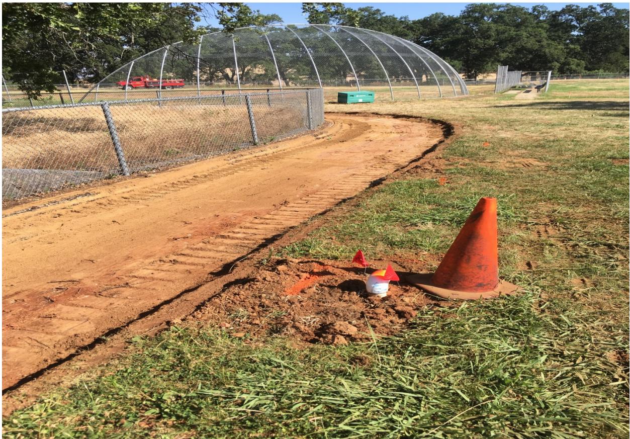
Track and Irrigation Install
