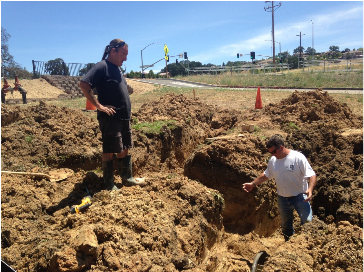
Chad and Duke Fixing One of Five Major Water Breaks
