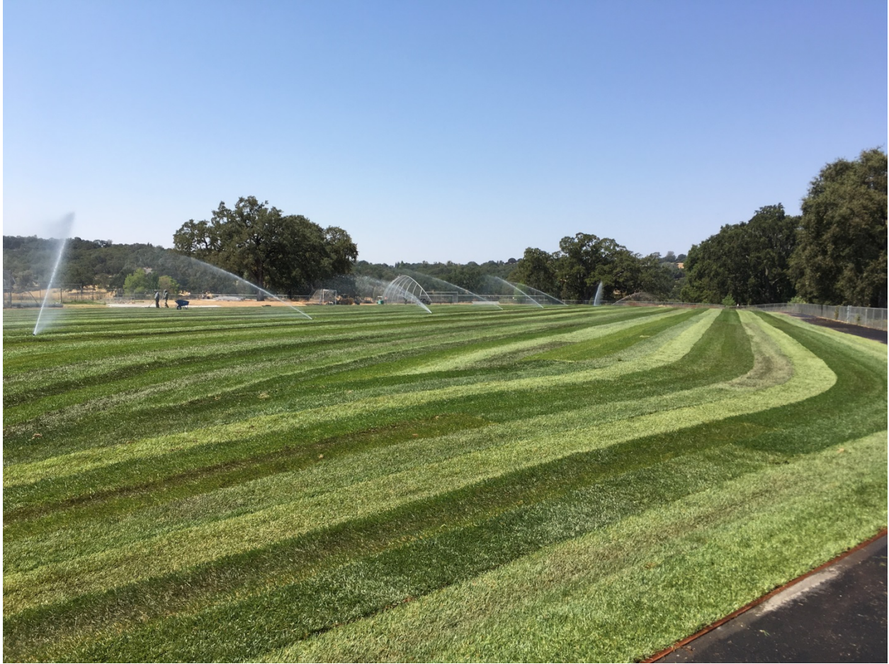
Track, Turf and Irrigation Project
