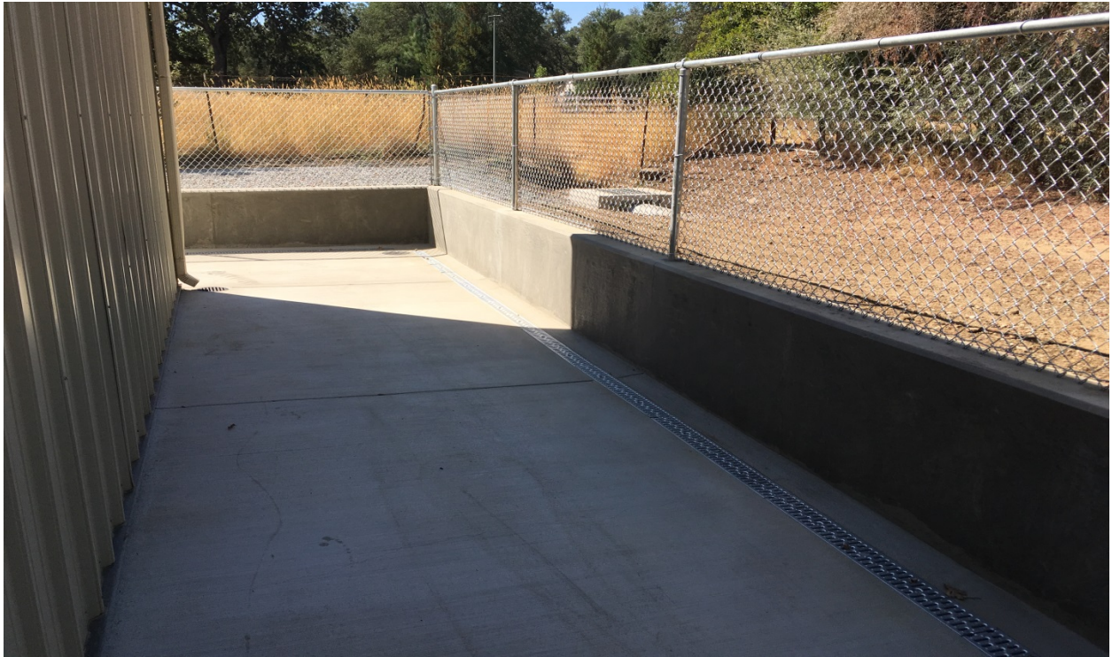
New Retaining Wall & Drainage Improvements
