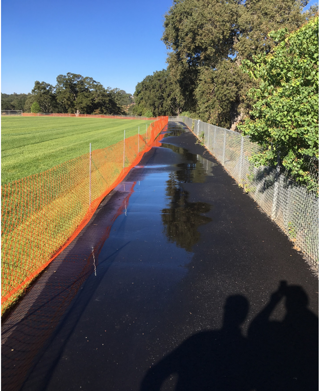
Track and Turf Install
